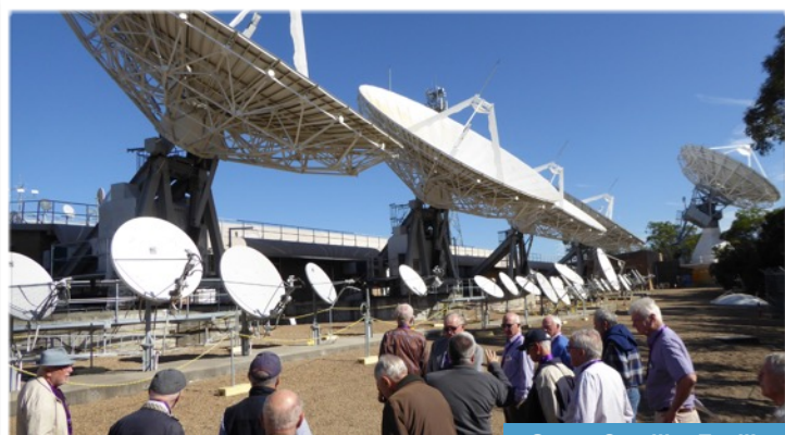
Optus Satellite Facility
